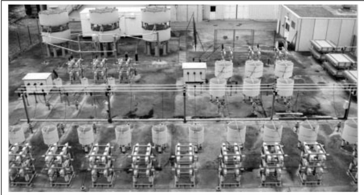
**Fig. 5:** Static Var Compensator based on Thyristor Controlled Reactor technology [2].
