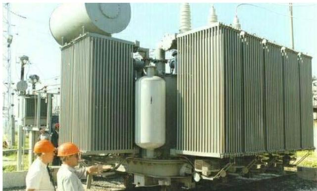
PermEnergo dramatically improved their system stability and gained from power savings when it installed this 3-phase, 25 Mvar, 110 kV, magnetically controlled shunt reactor at its Kudymkar Substation in NE European Russia in addition to an existing 3-phase, 32 Mvar, 110 kV shunt capacitor bank.
