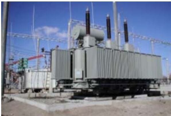
MCR 100 Mvar, 220 kV, E. Siberia, Russia
