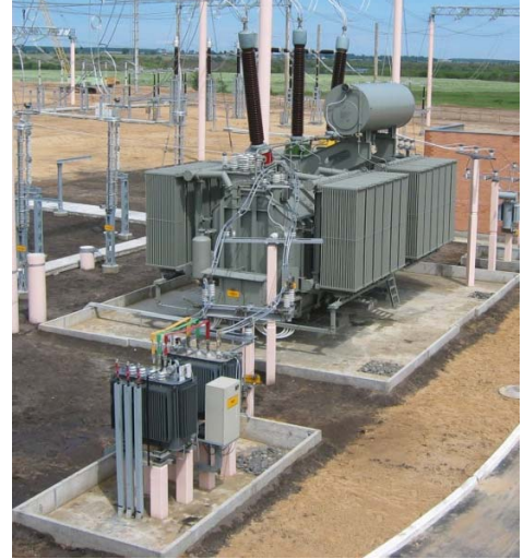
MCR 180 Mvar, 330 kV, Belarus
